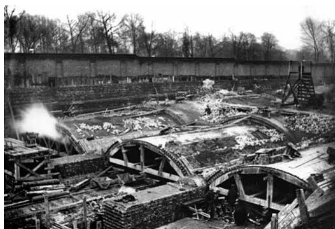
The photograph shows the construction work in progress. The tunnels were built by cut-and-cover. When finished, the area was covered over and the new cricket pitch laid.
